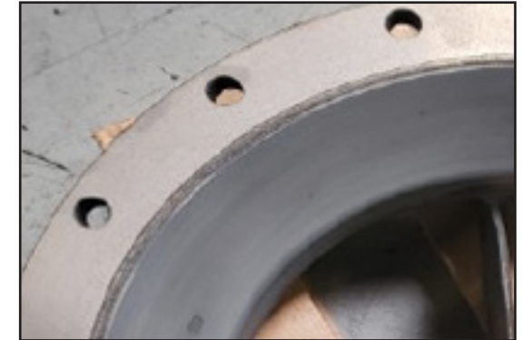
Suction bell successfully repaired with ARC 858 .
