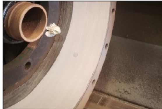
Suction bell being machined after ARC 858 was applied.
